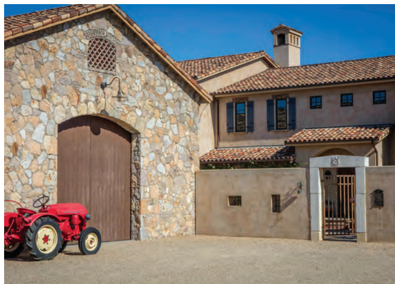
Renovations have begun on the winery paving the way for Krupp Brothers wine to be made at the new facility. ☞
